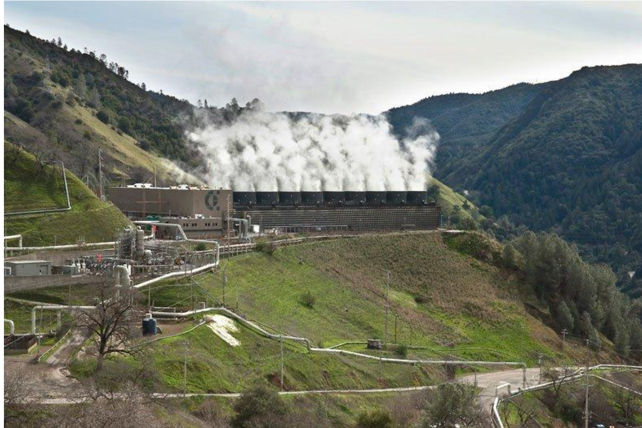
The Geysers (California). Dry steam. 250°C 20 units. Installed capacity 1400 MW Recharge of the reservoir with treated municipal waste water.
