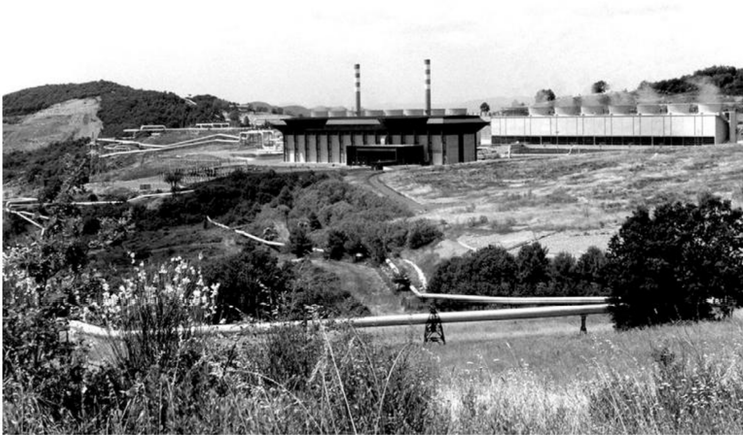
Valle Secolo geothermal power plant, Larderello, Italy; photo courtesy of Enel Green Power.
