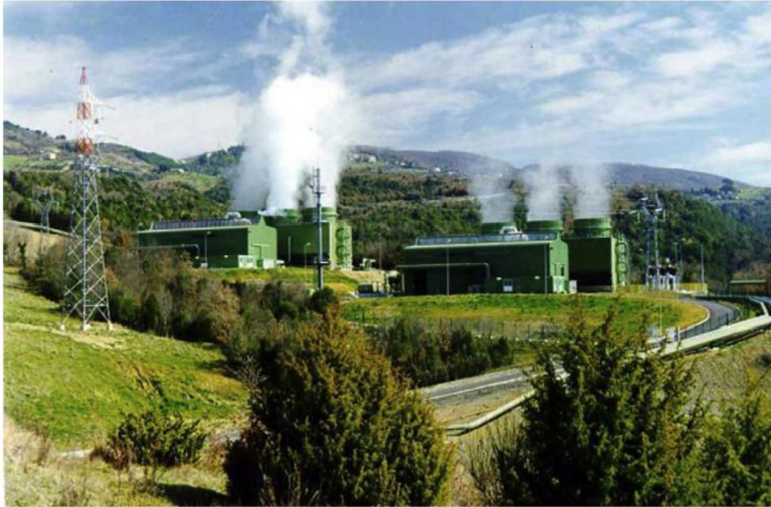
Figure 11.17 Carboli 2 \times 20 MW power units. Photo courtesy of ENEL Green Power [WWW].
