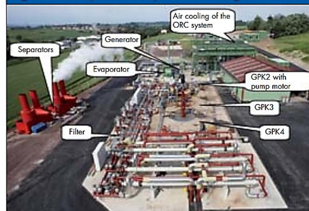
Fig. 9: Power plant and systems above ground
