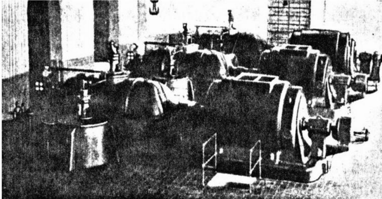
Figure 11.9 Three 2.5 MW steam turbine-generator units at Larderello, c. 1916 [11].
