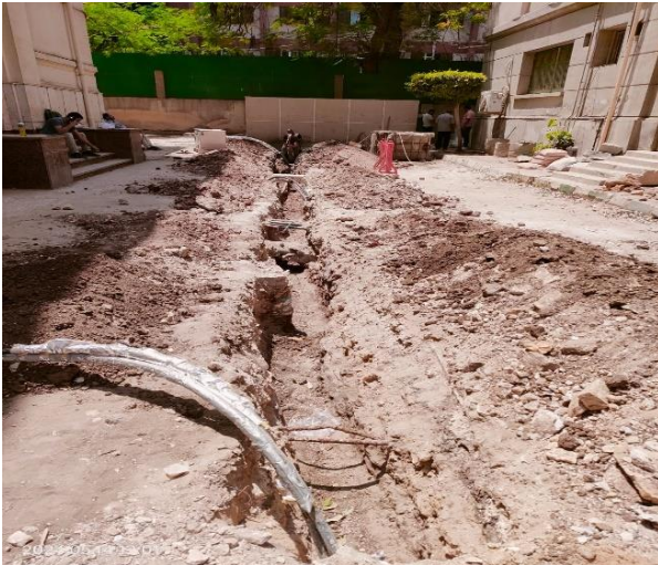
“Horizontal Trench for the three BHEs”
