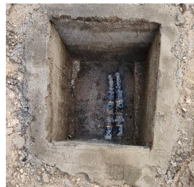
“Manhole constructed at BHE1”
