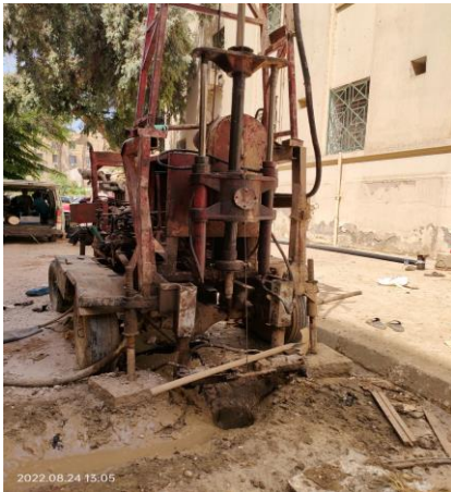
Exploration borehole at Faculty of Engineering- Cairo University
